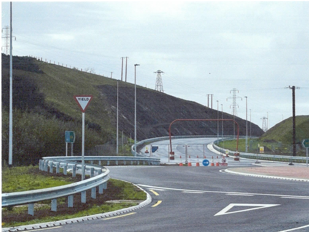
Plate 3 Western end of M28 cut through the Eastern end of the site
