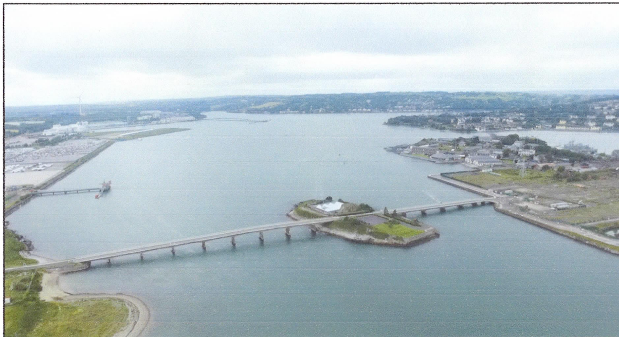
Plate 8 Aerial view towards the Naval College and the bridge across which 1000 naval personnel are expected to evacuate from Haulbowline Naval HQ
